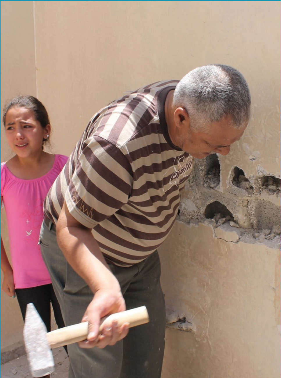
Self-demolition of a house in Jerusalem- Source: Al-Hadaf News Portal
